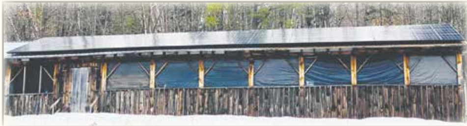
The 21.7kW DC rooftop solar array with 66 Hanwha modules and an Enphase microinverter system was installed by Southern Vermont Solar at Camp W's dining hall. It provides all of the camp's electrical needs. (Photos: Camp W)
