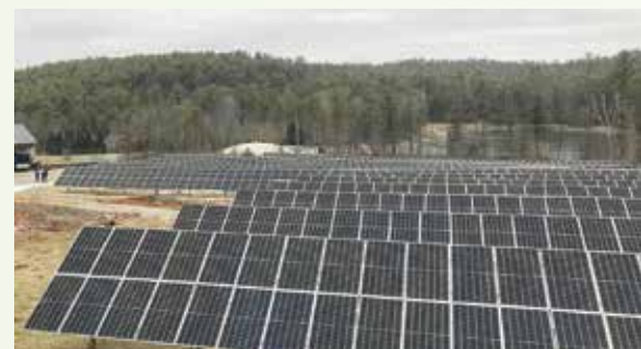
The first of two solar installation for Hanover, NH on Grasse Road. This 702kW installation is phase 1. Phase 2 community solar on this site will accommodate a 1021kW system. Image: Sustainable Hanover.
