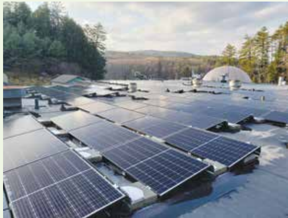
A 68 kW solar system at the Water Reclamation Facility in Hanover. Images courtesy of Sustainable Hanover, unless otherwise noted.
