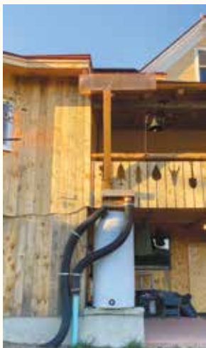
Rainwater catchment system on Kroka's new farmhouse.
